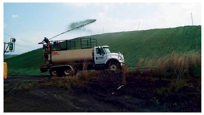
Hydraulic erosion control products are applied as a slurry and engineered to reduce soil erosion while assisting in the establishment and growth of vegetation.
